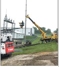
the transmission line into the substation is being replaced. Inside the substation, CRMU will be replacing the gang-operated air-break switches, the fused knife switches, along with installing a new secondary riser structure and metering cabinet.
